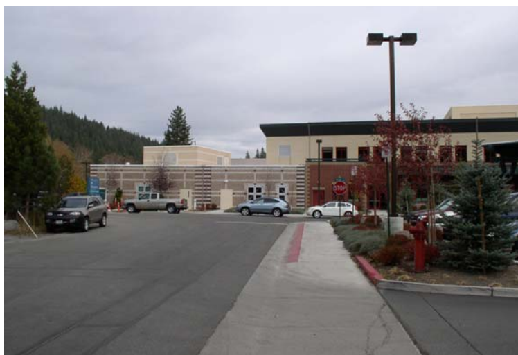
View from Tahoe Drive - Looking East toward Pine Avenue at the Northwest corner of the existing Tahoe Forest Hospital
