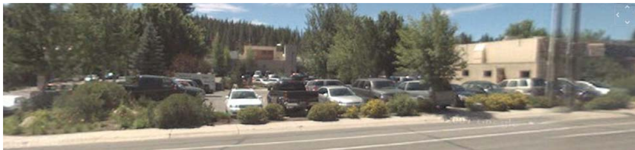
Existing view of Tahoe Forest Hospital from Donner Pass Road
