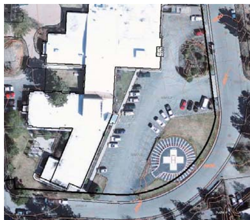
Existing Heliport Pad
